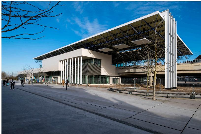
The station building received a thorough makeover. One part was demolished and replaced by a new building, another part was dismantled and renovated. Under the existing railway viaduct, we installed 2,500 m<sup>2</sup> of waterproof ceiling, and above the tracks and the station we mounted a new canopy. During the works, the station remained in service as usual.
