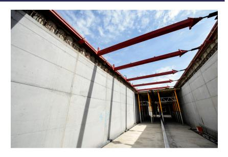
Storm water reservoirs connected to the drainage system that can collect  $10,000~\text{m}^3$  of water during heavy storms, relieving the pressure on sewers. Buffered water is discharged into one of the main collectors in Brussels, half using a gravitational outlet, the other half using pumps.
