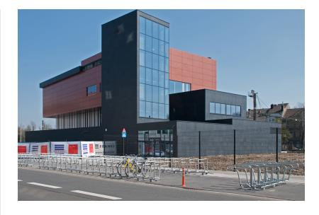
Construction of a signalling centre for the Belgian railways and demolition of an existing post office building. The complete building forms a Faraday cage to protect the railway signalling. This was accomplished by earthing 4,100 m<sup>2</sup> of concrete walls and interconnecting all concrete reinforcement.
