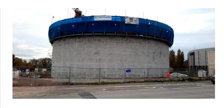
Construction of a cylindrical concrete drinking water reservoir with an inner diameter of 38.4 m, a wall (via sliding formwork) with a thickness of 45 cm and a height of 16.5 m, including surrounding construction.
