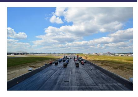
During the summer of 2020, Willemen Infra was responsible for the renovation works on runway 07L/25R at Brussels Airport. The works were delivered on time. For six weeks, work was carried out around the clock 7 days a week to limit the duration of the runway closure and the impact of these works. The thorough renovation of this runway was necessary to guarantee the safety of air traffic in the future.
