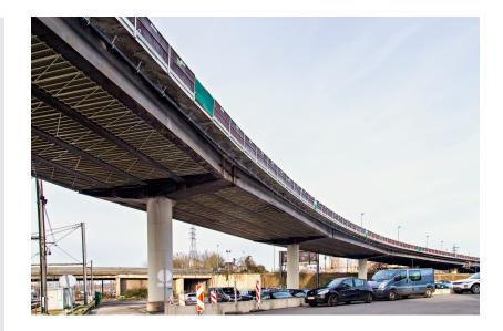
Public works contract for the complete reconstruction of the southern part of the Charleroi R9 ringroad, (1, 670 m + 2 x 400 m of A503 sliproads), on both the upper and lower faces of the viaduct section, while maintaining traffic circulation.
