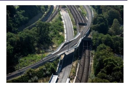
The project consisted of infrastructure work along the track bed platform where railway lines L124 and L26 intersect. Several bridge decks were renovated and noise barriers installed, including 2,000 m<sup>2</sup> of green walls. For the Moensberg station at Uccle, new platforms have been built. Simultaneous with these main works diverse road, bedding, demolition, earth- and sewerage works were performed.
