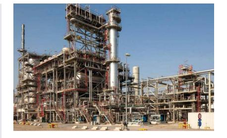
This project was part of a worldwide effort to expand and modify three refineries in Europe (including Antwerp) and the US to produce cleaner diesel. This increased the production of low sulfur diesel in these plants by over 22 million litres per day. The High Pressure Hydrotreater is a system that desulfurises diesel with hydrogen under high pressure.
