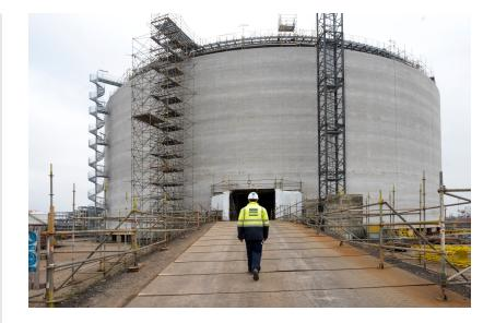
Franki Construct built an ammonia tank on the BASF site in the port of Antwerp for the German petroleum & gas engineering company, SPG Steiner. The tank's diameter is 72 m, and it is more than 26 m high. The 26-m high concrete wall was erected in a continuous 24-hour shift system using sliding formwork.
