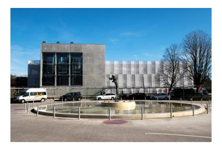
For Antwerp University Hospital, we built a brand-new 27,000 m<sup>2</sup> visitor car park with 960 spaces spread over four floors. The car park consists of a prefabricated concrete structure and is equipped with an intelligent parking system. Thanks to extensive LEAN planning, we were able to deliver the project ready for use in less than 8 months.
