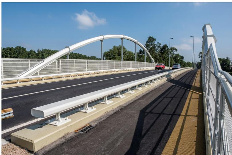
The project involves replacing the arch bridge over Moerbrugsestraat in Oostkamp, widening the bridge over the River Brook and adapting the Moerbrugsestraat road alignment between Rivierstraat and Stationsstraat. The new arch bridge consists of two lanes for motorised traffic and a cycle path along both sides.
