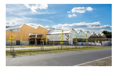
Oh'Green's new site in Aarschot is a pilot shop of Garden Center Holding. Cosimco was responsible for its construction on a site of just over 44,000 m<sup>2</sup>. Due to the conditions imposed by the PRUP, the building was designed lengthwise, parallel to the Diestsesteenweg. Due to the steeply sloping terrain in the first 50 metres from the street, the garden centre was built half underground.
