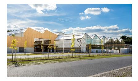
Oh'Green's new site in Aarschot is a pilot shop of Garden Center Holding. Cosimco was responsible for its construction on a site of just over 44,000 m<sup>2</sup>. Due to the conditions imposed by the PRUP, the building was designed lengthwise, parallel to the Diestsesteenweg. Due to the steeply sloping terrain in the first 50 metres from the street, the garden centre was built half underground.
