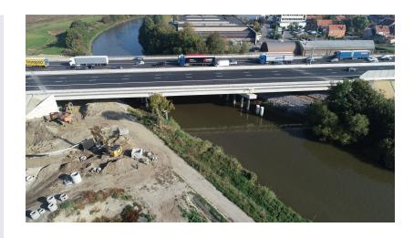
In Merelbeke, two bridges on the E40 were renewed and widened, and adapted to much heavier (exceptional) traffic: the bridge over the Tijarm (a tributary of the Scheldt) and the bridge over the Oude Gaversesteenweg. A temporary bridge ensured that traffic on the E40 remained possible in both directions during the works.
