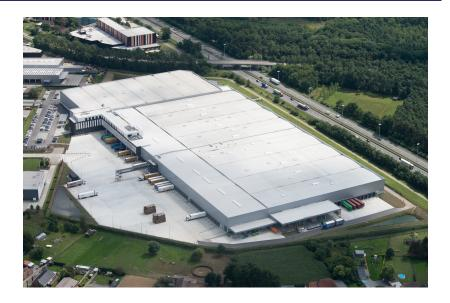
On a site of just over 10 hectares along the E313 motorway, we built a  $50,000 \, \text{m}^2$  distribution centre with 62 loading docks. From this location, CASA shops have been supplied throughout Europe since 2017. Thanks to a space that can accommodate 65,000 pallets, the company can save 5,000 freight trips a year. In addition to the warehouse and the necessary technical areas, the new building comprises  $5,000 \, \text{m}^2$  of offices spread over four floors.
